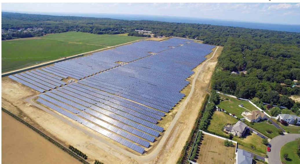
Borrego's 14.3 MW sPower Shoreham solar project in Suffolk County, Long Island.
