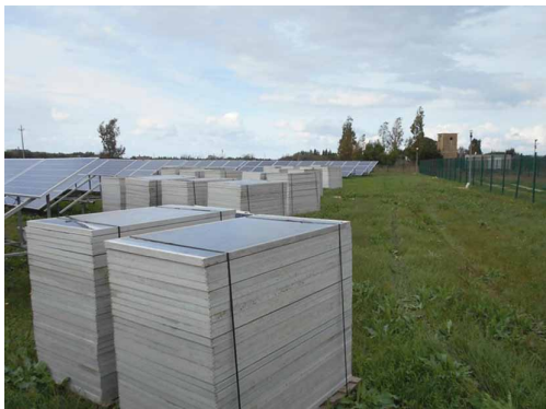
A PV plant in Italy in the process of revamping, following six years of service.
